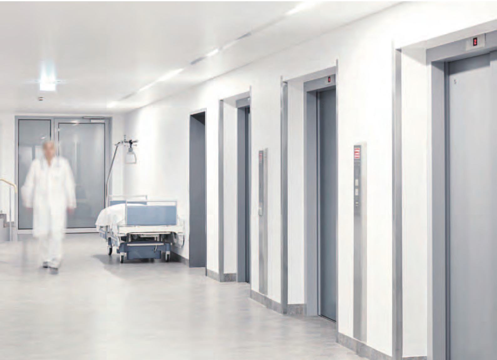
A TYPICAL COMMERCIAL ELEVATOR USED IN HOSPITALS
