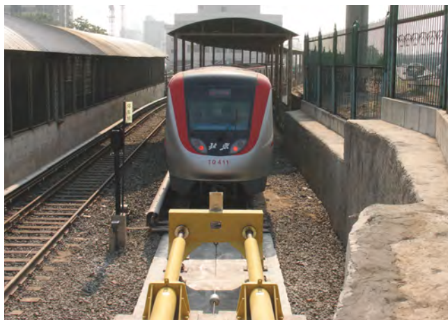
Typically used on metro and main lines – designed for centre and side impact. Concrete base foundation incorporating Oleo hydraulic units (two Oleo Type 730 – Recoverable stroke 3000mm). Train mass: 510 tonnes, Impacting speed: 12km/h, Installation length: 9.5metres, Impact capacity 3360kj.
