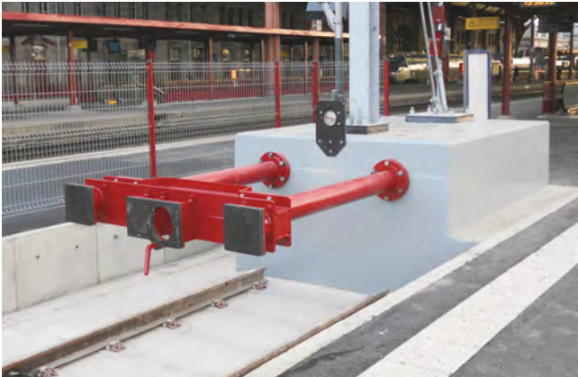
Typically used on metro and main line – designed for centre and side impact. Concrete base foundation incorporating Oleo hydraulic units (two Oleo Type 718 – Recoverable stroke: 1800mm). Train mass: 267 tonnes, Impacting speed: 12km/h, Impact capacity: 2016kj, Installation length: 5.5m.
