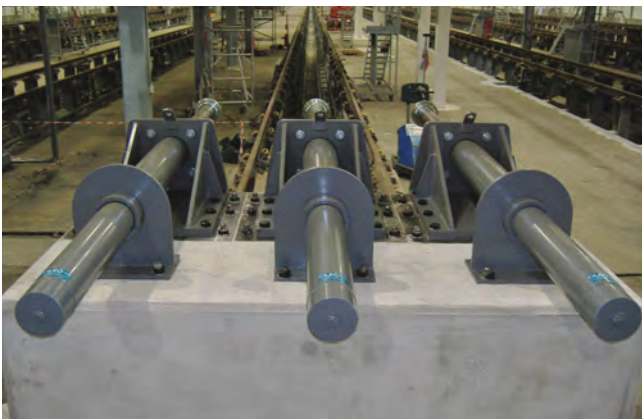
Typically used on metro, main line and depots – designed for centre and side impact. Concrete base foundation incorporating Oleo hydraulic units (three Oleo Type 712 – Recoverable stroke: 1200mm). Train mass: 1000 tonnes, Impacting speed: 1.94m/s, Impact capacity 2016kj, Installation length: 3.5m.
