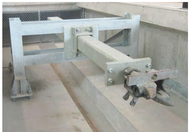
This project involved the client designing their own steel structure which was mounted onto a concrete base. Designed for centre impact incorporating Oleo hydraulic units (two Oleo Type 76 units – Recoverable stroke 1200mm). Train mass: 115 tonnes, Impacting speed: 8km/h, Installation length: 3.5metres, Impact capacity 672kj, End force: 700kN.
